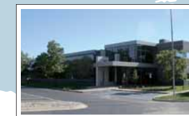
Continental Structural Plastics Holdings Corporation
